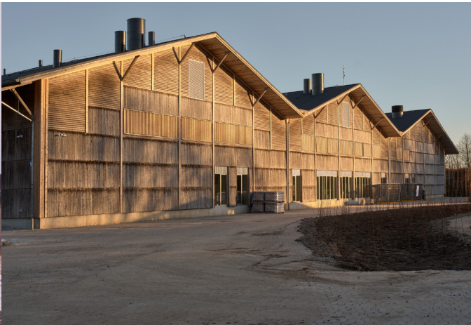
Rear façade, before and after refurbishment. The modular panels allow new elements to be inserted wherever required with ease. The first-floor windows are concealed behind timber slats.
